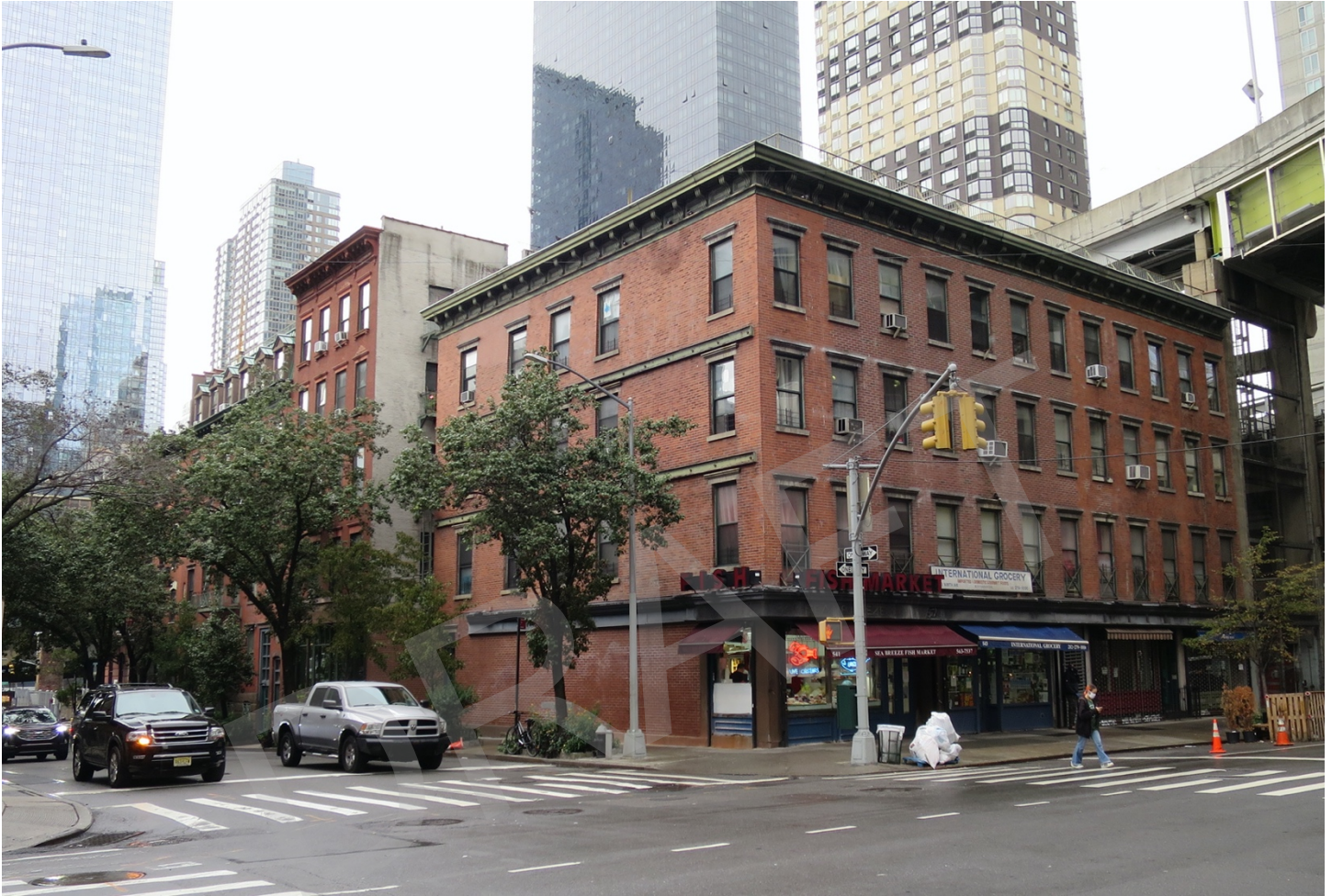
Image 15: View of the northeast corner of Ninth Avenue and West 40th Street.
