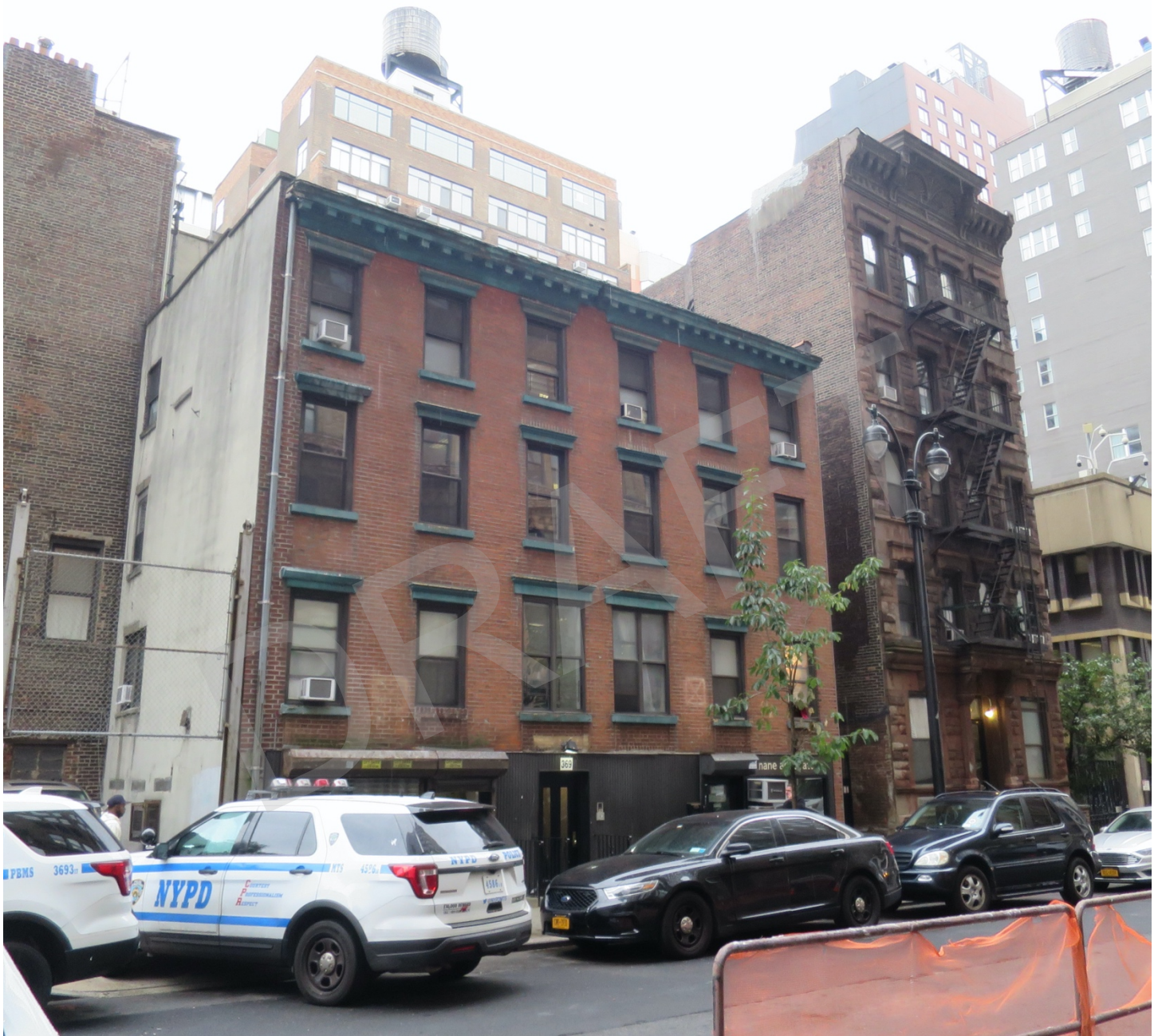
Image 1: View of north side of West 35th Street, east of Ninth Avenue.
