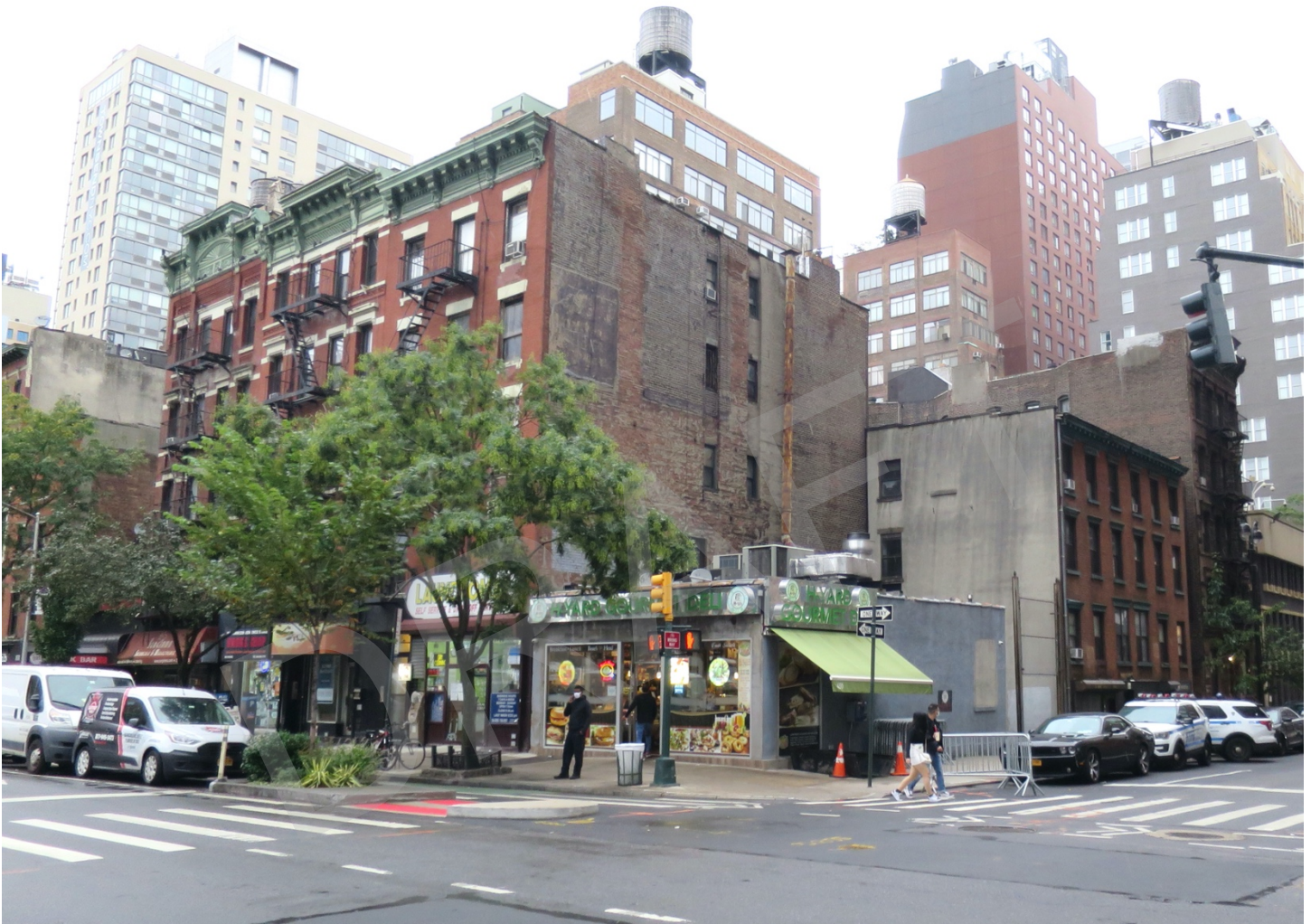
Image 2: View of the northeast corner of Ninth Avenue and West 35th Street.
